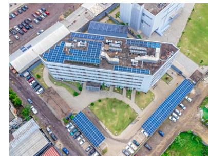
Solar system for a technical building of our customer, Aktivco SaaS project - Cameroon
