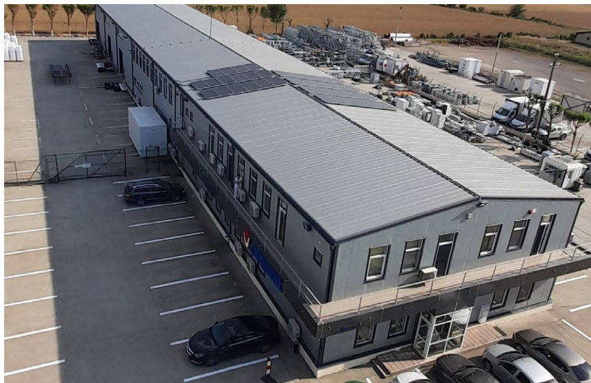
Solar panels on our administrative building - Romania
